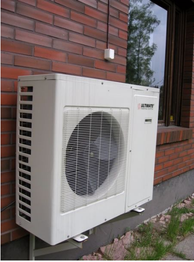
Figure 13-3: External heat exchanger of an air source heat pump for heating and cooling of a residential building. Wikimedia commons
